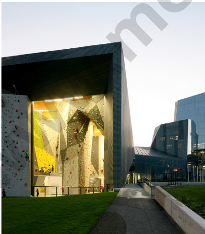
Salewa Headquarters, Bolzano/Italy (2007-2011)
