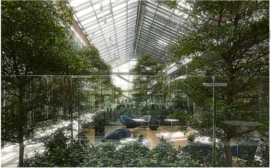
Prysmian Group Headquarters, Milano/Italy (2014-2017)
